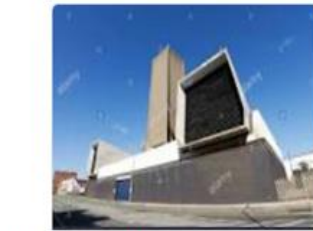
Liverpool Ventilation Shaft
