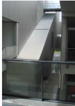
Fig. 15 Staircase 'bolted on'
